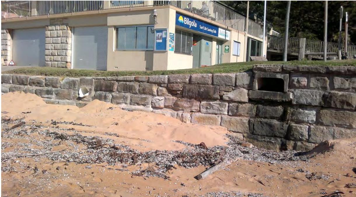
**Figure A16: View of sandstone block seawall seaward of Bilgola SLSC, 4 June 2015**
