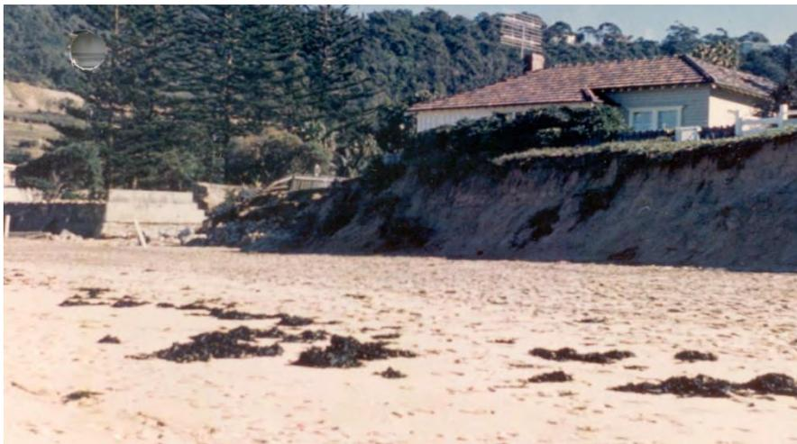
**Figure A1: Dune erosion at Bilgola Beach after June 1966 storm (derived from Wilson, 1966), with 21 Bilgola Avenue seawall evident on left hand side**
