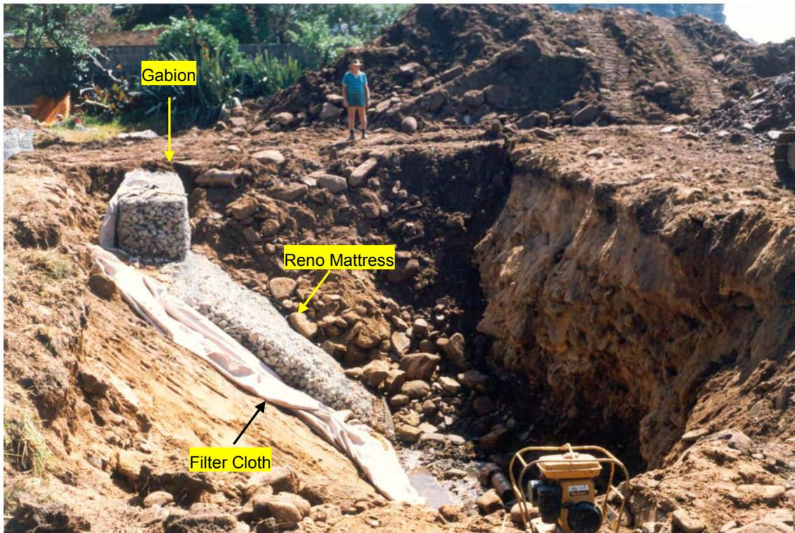
**Figure A15: Gabion revetment under construction at 21 Bilgola Avenue in October 1993**
