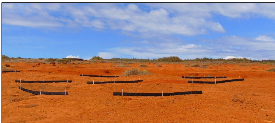
Figure 24 ProWattle™ installed above the CIP Project site in 2019
