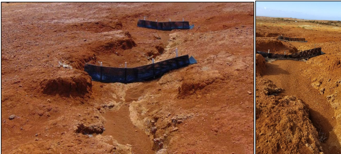
Figure 26a, b Ditch Guard™ installation in Kamōhio Watershed
