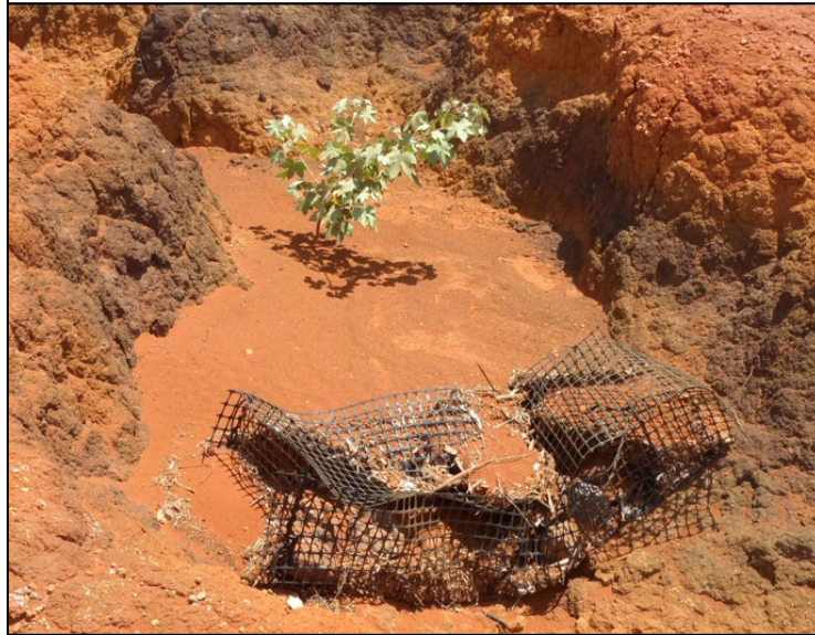
Figure 37 Silt captured behind a gabion with a Hawaiian cotton (Ma'o) plant
