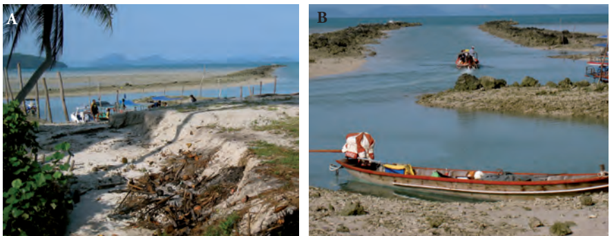
● Fig. 34. Drainage canals, not only on the terrestrial parts (A), but also in the coastal intertidal and subtidal coral (rubble) platform to allow the long-tail boats to get close to the beaches for the tourists, even at low tide (B).
