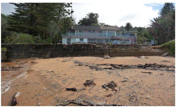
Figure A12: Vertical seawall at 21 Bilgola Avenue, partially exposed after storms on 22 April 2015
