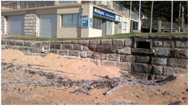
Figure A16: View of sandstone block seawall seaward of Bilgola SLSC, 4 June 2015
