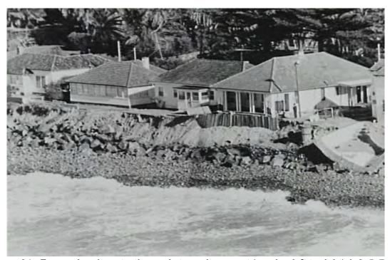
Figure A4: Exposed rock protection and storm damage at (moving left to right) 1, 3, 5, 7 and 9 Allen Avenue (with undermined swimming pool at latter), 28 May 1974
