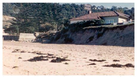
Figure A1: Dune erosion at Bilgola Beach after June 1966 storm (derived from Wilson, 1966), with 21 Bilgola Avenue seawall evident on left hand side
