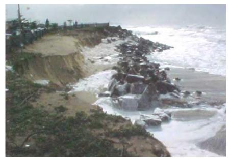
Figure D17: Erosion landward of revetment at Stockton Beach in July 1999
