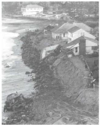
Figure A9: View looking south of storm damage and rock protection at Bilgola Beach on 11June 1974 (from PWD, 1985)
