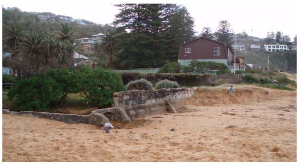
Figure A11: Vertical seawall at 21 Bilgola Avenue, partially exposed after storms on 21 July 2007
