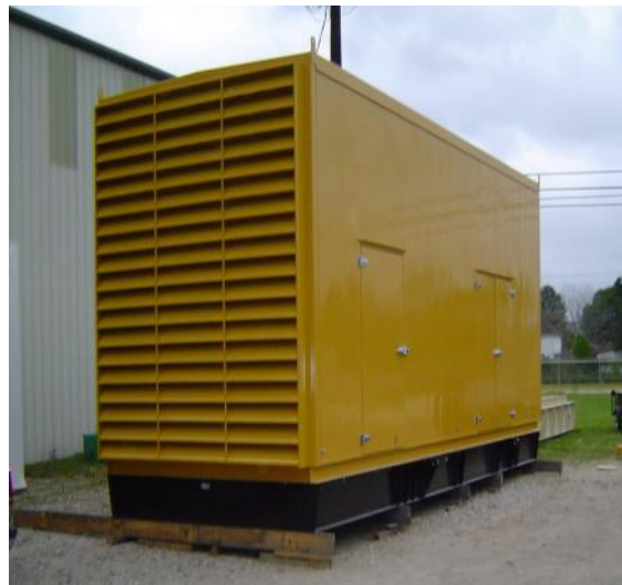
Plate b. Generator sound attenuation house
