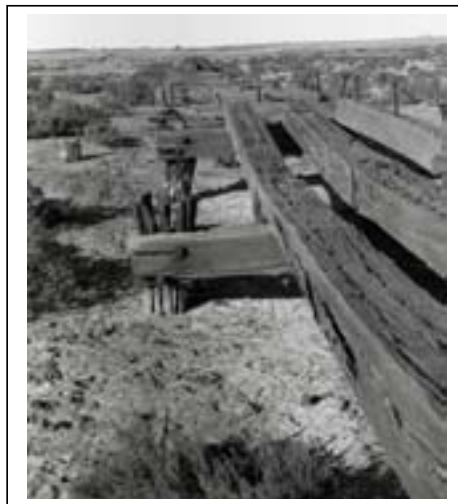
Figure 4 1991 photograph of large timber bridge over tidal flats
