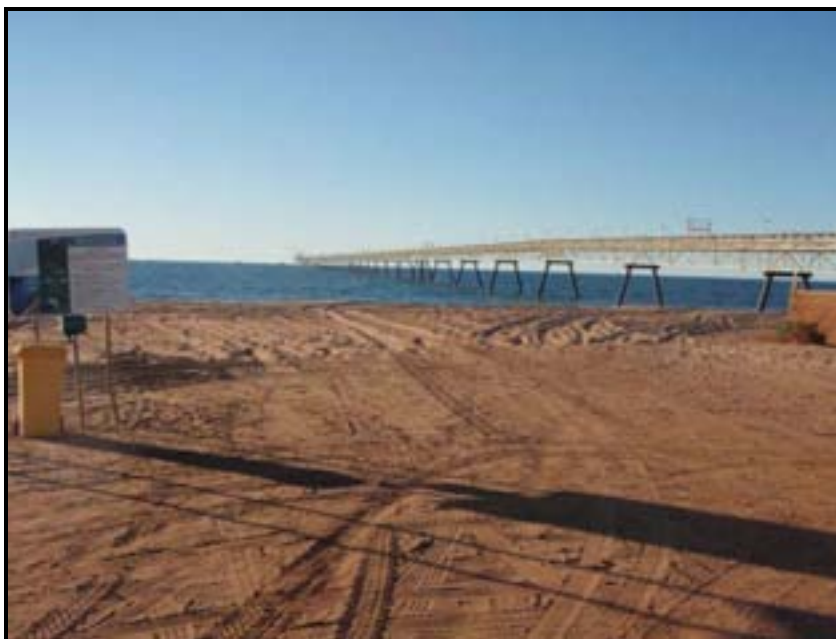
Photograph 2.1: An example of wide spaced pile bents (Onslow Salt jetty).
