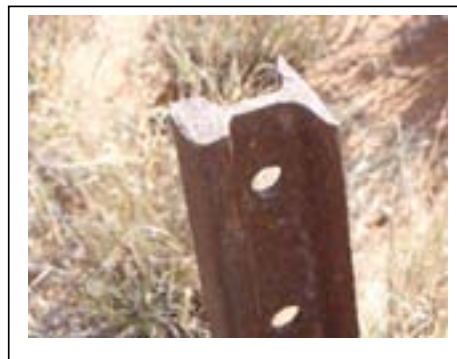
Figure 25 Tram rail used as fence post
