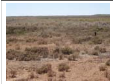
Figure 31 Telegraph pole base
