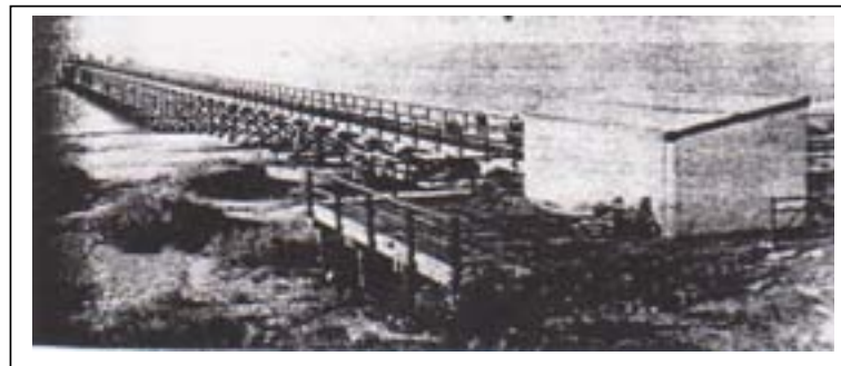
Figure 5 Historic photograph of sea jetty showing timber platform in dune system
