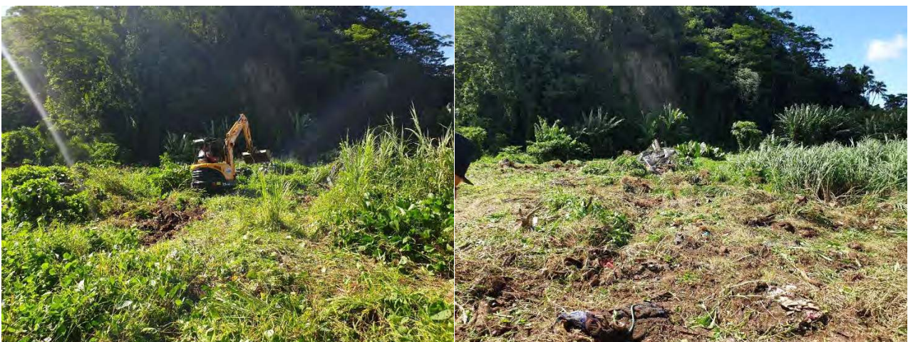
Figure 6 Site before and after clearance
