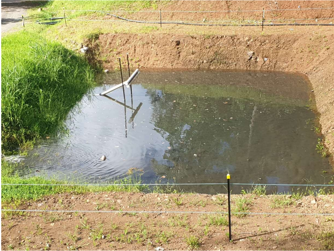
Figure 11 – Ngatoe scour pond
