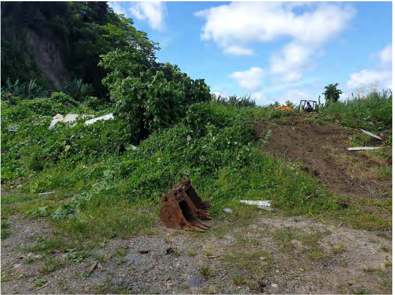
Figure 5 Site 88H fill Platform
