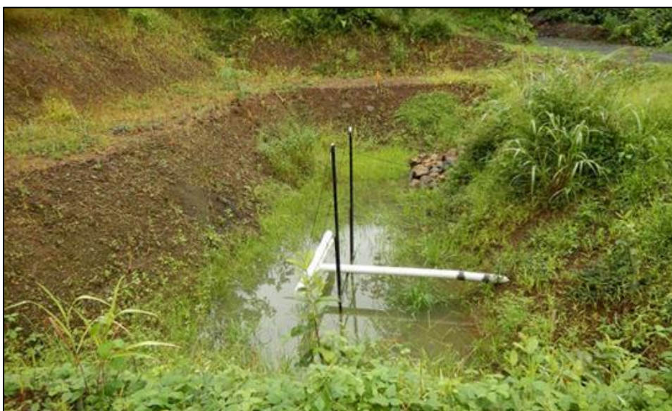
Figure 5.3: Photo of a settling pond showing the two compartments, at the Avana Water Treatment Plant.
