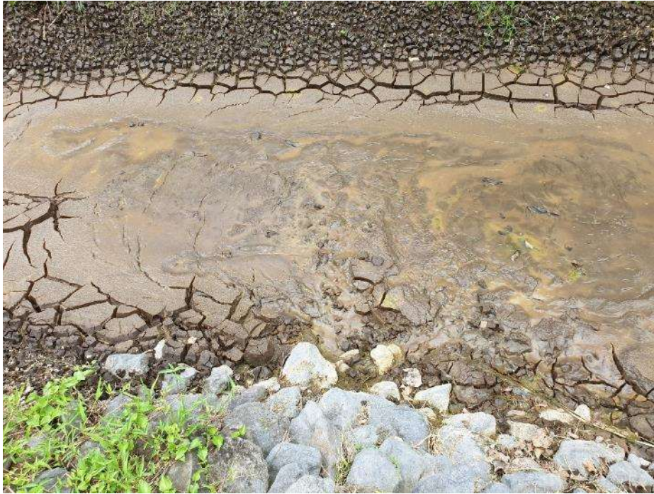
Figure 19 - Matavera pond approximately two days after discharging settling tank residuals (1 Feb 2021). The pond is in standby (drying) mode.
