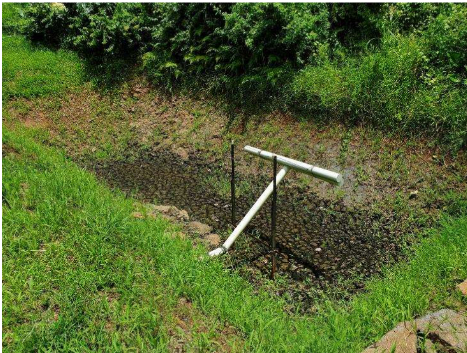
Figure 20 - Tupapa upstream (standby) pond on 11 Feb 2021
