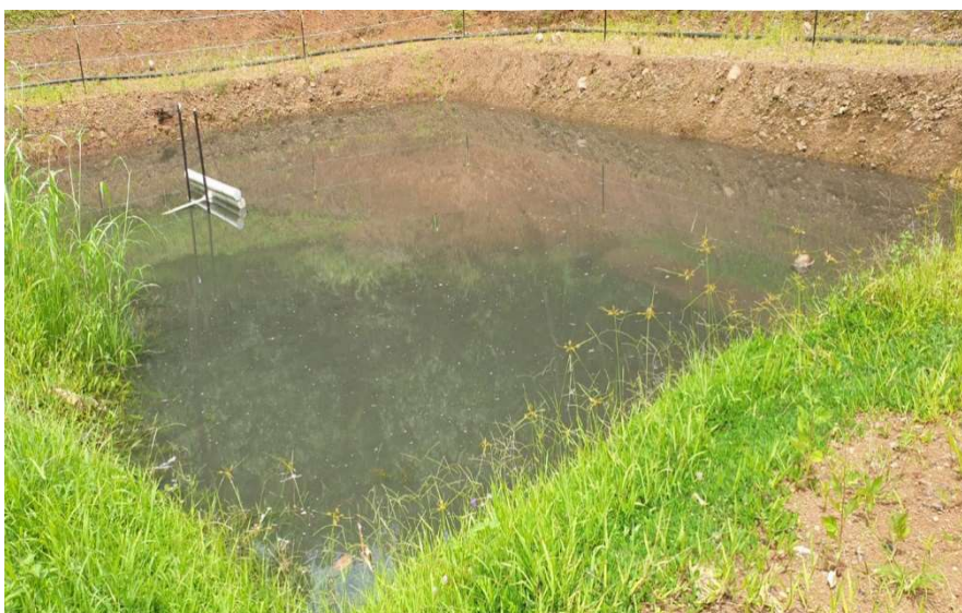
Figure 12 – Ngatoe scour pond after desludging (2 Dec 2020)
