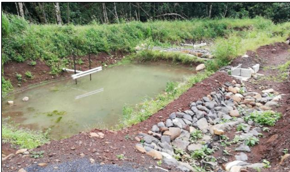
Figure 5.2: Scour pond on the Ngatote catchment.
