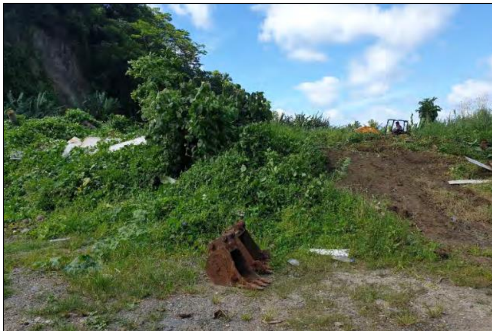
Figure 4.4: Site 88H fill platform
